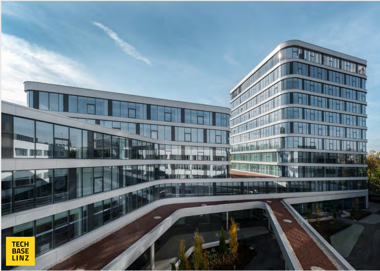
Lessees building section 2: Agilox, BDO Upper Austria, Siemens Upper Austria, Siemens Healthineers, Wiesner Hager Lessees building section 1: Apleona, Humanetics, Industrie Informatik, Yunex Traffic
