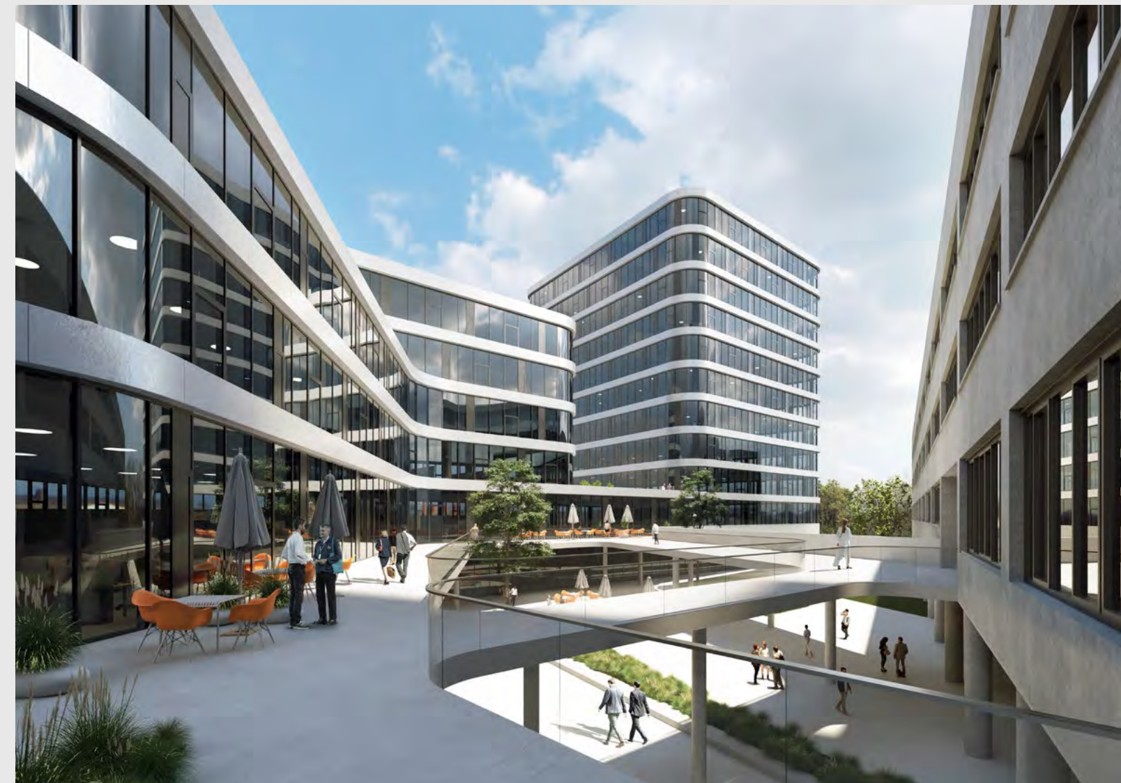
Catering, shops and recreational areas: A generous range of facilities create open spaces for companies and their employees to meet and relax.
